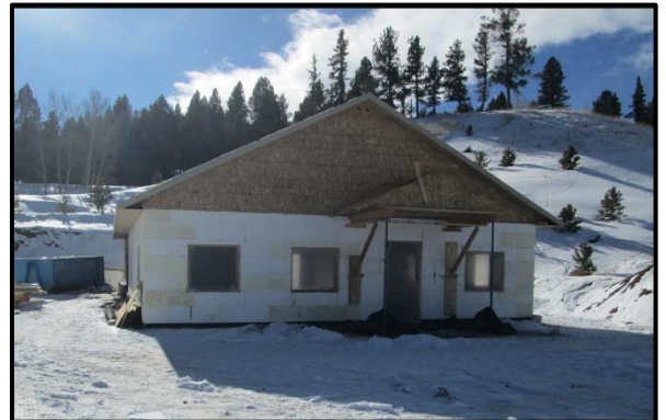
MMWC new office under construction.
